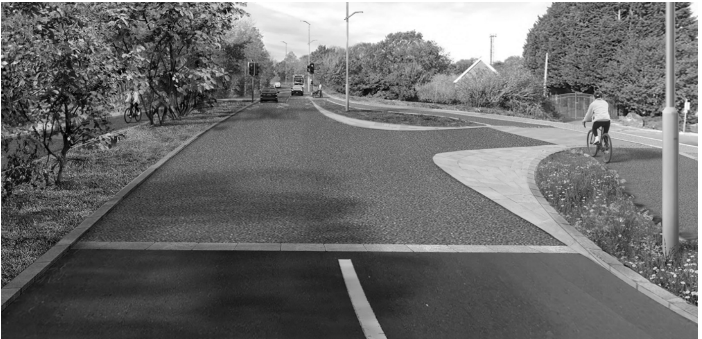
Change to surface treatments and corner radii slow vehicle speeds, along Baldock Road (A507) with access to the Buntingford Business Park. .
